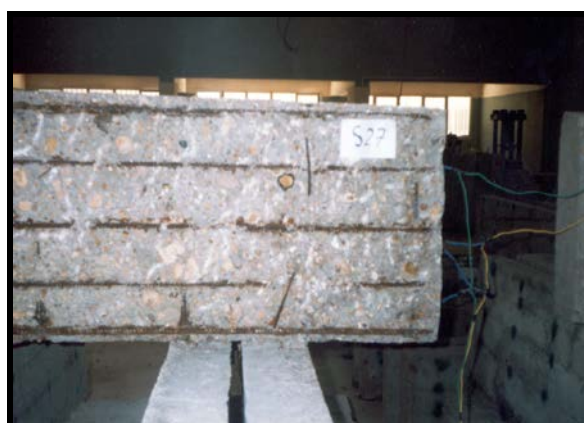
Fig. (1 a) Removing of contaminated concrete covered layer of slab27 (M).
