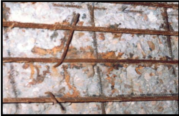
Fig. (1 b) Removing of contaminated concrete covered layer of slab27 (H).
